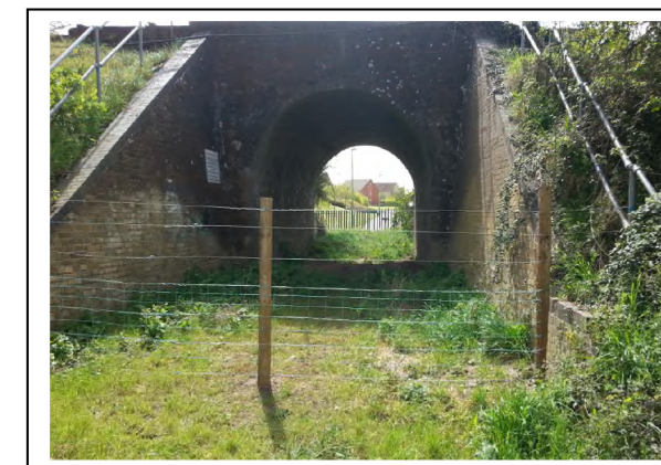
Photo 2: Alternative railway crossing - underpass
